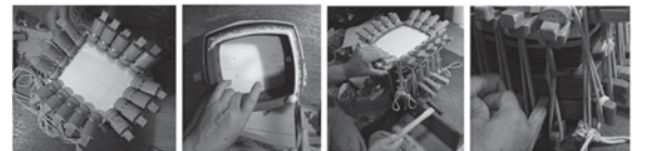
Attachment of the wooden pins Attachment of the bond to the wooden frame Under tension by wooden wedge Control of the tension with tapping by the nail
