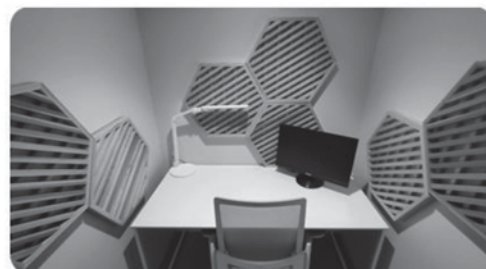
Fig. 1: room B-CRD diffusion type installed
