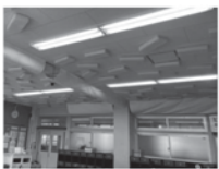
Fig.1: The classroom with sound absorbing materials
